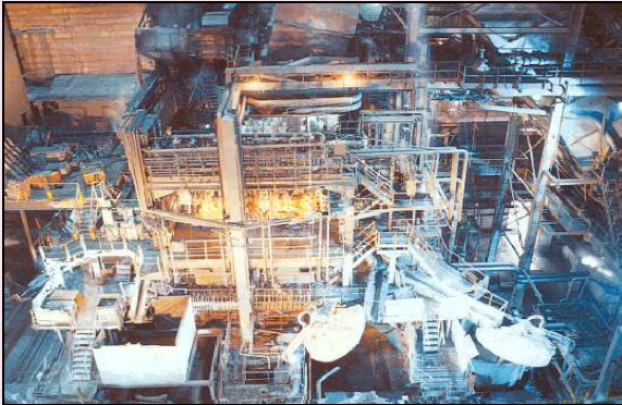
The Romelt furnace under operation
